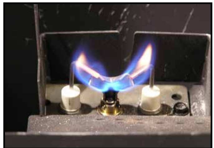
Figure 4.1 IPI Pilot Flame Pattern
