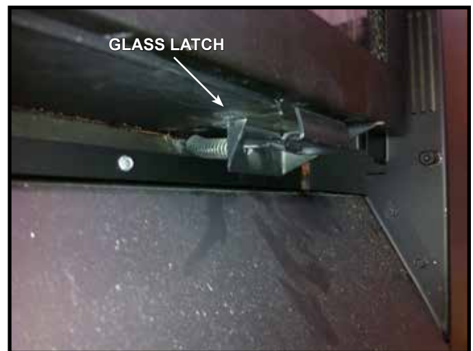
4.4 Glass Latch Detail - Exterior Side
